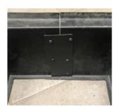
**2** Core drill lid at riser position. Use cutting tool to slot lid. Blend lid into position.
